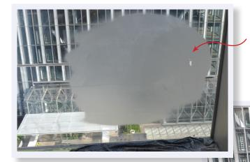
A glass panel showing almost the whole area flattened by abrasive slurry, there is only one small distortion remaining
